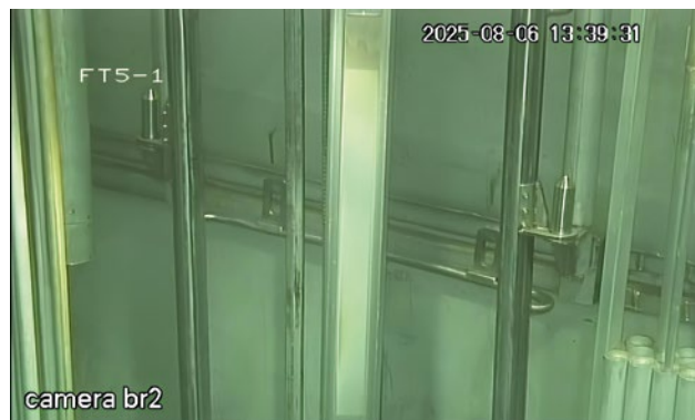
Figure 2: Visual inspection of one FUTURE-MONO-1 fuel plate in the BR2 reactor.
