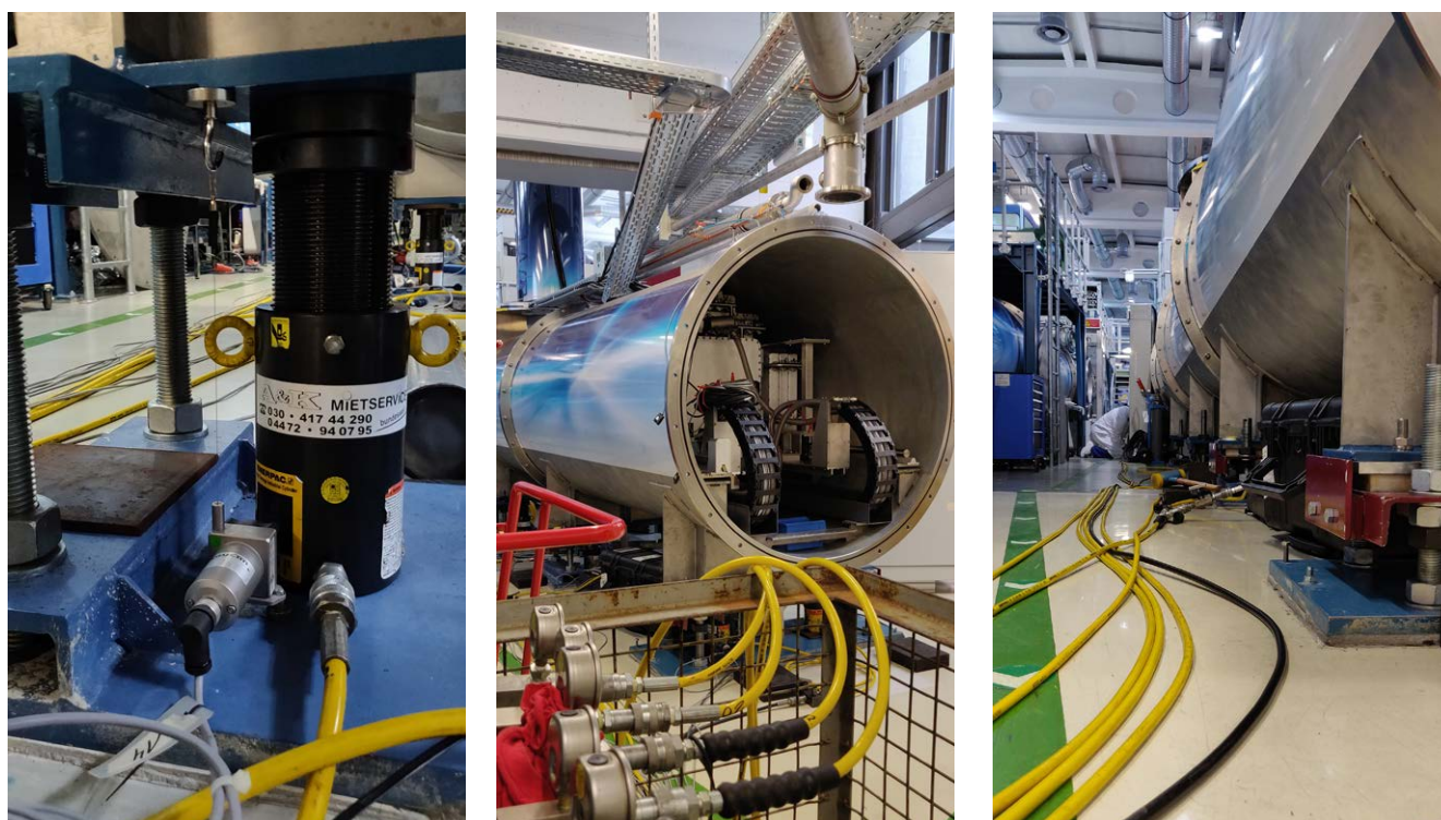
Figure 1: Hydraulic system positioned under the detector tube.
