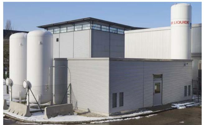
Fig. 2: Newly built housing to the south of the MLL for the He-compressors of the UCN-source, with two helium gas tanks (on the left) and a liquid nitrogen tank (on the right).
