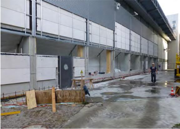
Figure 13: Preparation of the construction zone between the Experimental Hall and the new Neutron Guide Hall East with wall elements already deinstalled.
