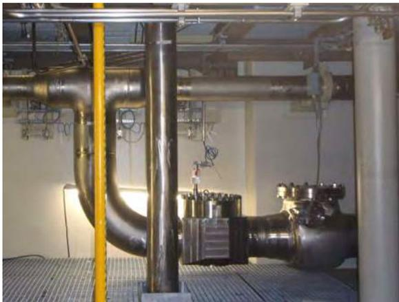
Figure 2: The two main check valves: the new one on the left, the original one on the right.
