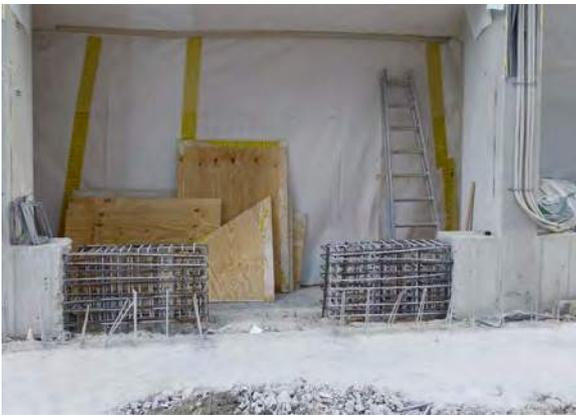
Figure 14: Removal and reconstruction of concrete base for provision of a new entrance from the Neutron Guide Hall East to the new building connecting the Experimental Hall and Neutron Guide Hall East.
