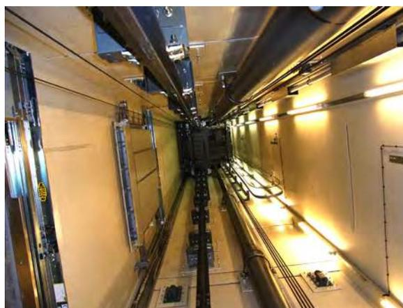
Figure 3: New freight elevator with a lifting capacity of 10 tons in the reactor building.
