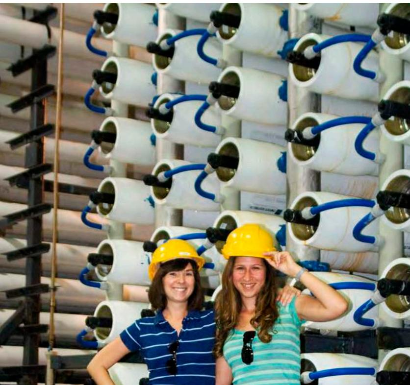
Figure 1: Ashkelon Seawater Desalination Plant (Israel) using Reverse Osmosis (RO) Technique. Produces 330,000 m<sup>3</sup> potable water per day for 0.57 \$/m<sup>3</sup>. The two young ladies are former students of the Zuckerberg Institute for Water Research.
