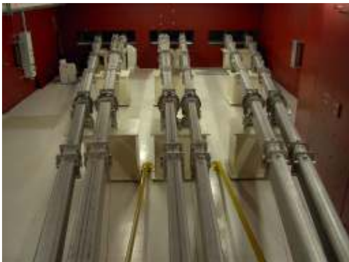
Figure 8.8: The 6 NG lines NL1 to NL6 passing through the tunnel area. Along the vacuum tubes joints, windows and adjustment elements are visible.
