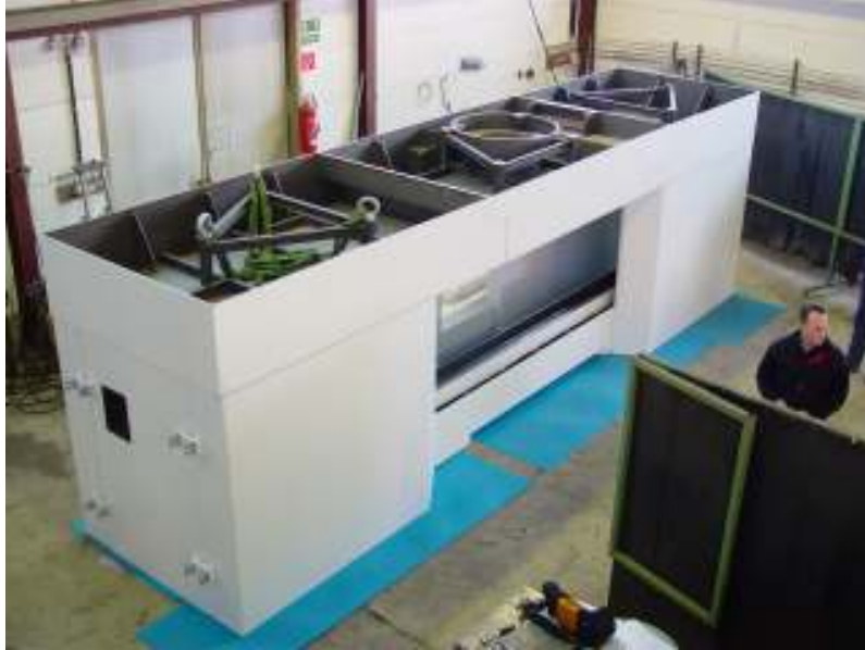
Figure 3.3: Monochromator shielding without sliding front wall during construction
