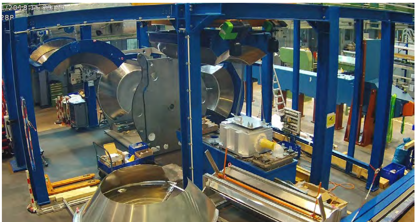
Figure 7: POWTEX takes shape in the ZEA-1 workshop area in Jülich.
