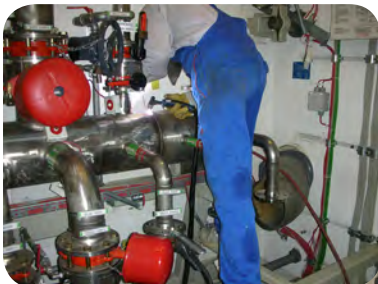
Working at the fitting.
